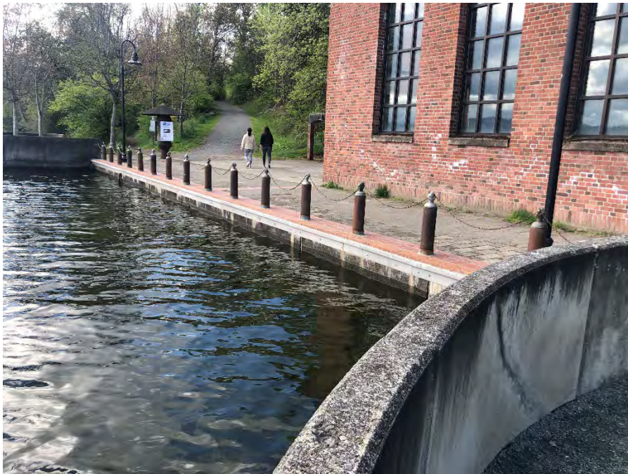
Photograph 4. Handsome Bollards chain and existing bulkhead in front of Boiler Building (April 2021).
